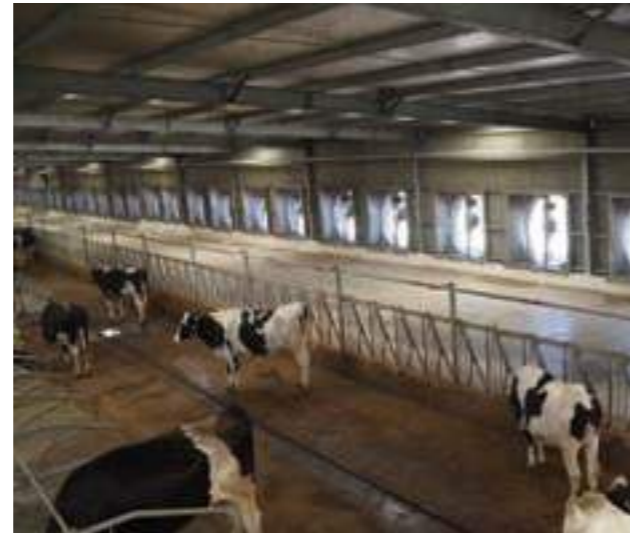
Automatically controlled cooling cowshed via THI
