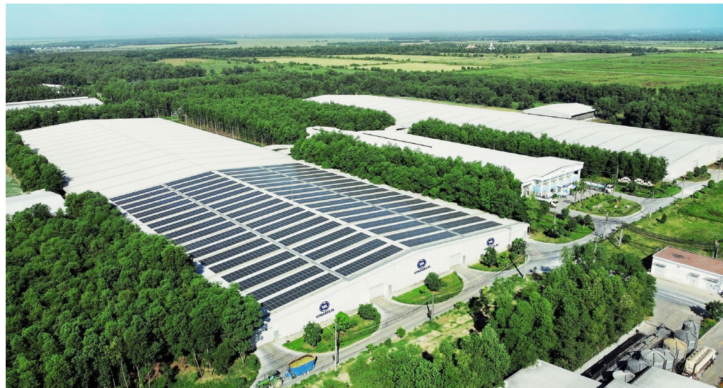
Solar panel installed on the roof of a farm
