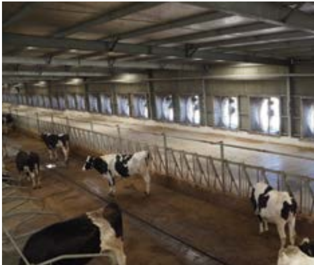
Automatically controlled cooling cowshed via THI
