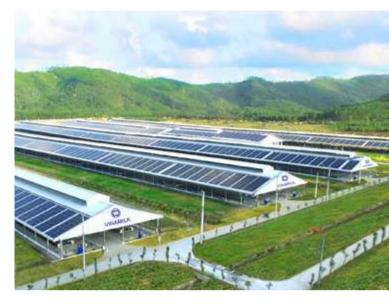
of cow barns in all of Vinamilk's dairy farms. By the end of 2020, solar panels have been installed in 05 farms: Binh Dinh (2.96 MWp), VNM Da Lat (2.06MWp), Organic (1.18MWp), Di Linh (0.99 MWp) and Quang Ngai, the last of which is still in progress, and it is expected that by June 2021, all the other farms in Vinamilk's system will have their own source of solar energy for consumption.
